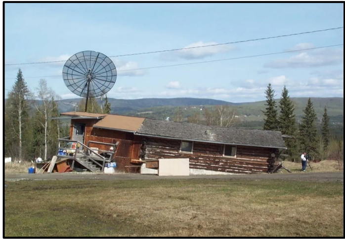
Figure 11: House sinking due to permafrost melting near Fairbanks, Alaska.
